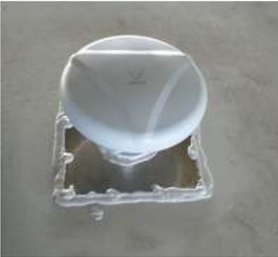
I removed the old motorized one, and configured a 12 inch square by 3/16<sup>th</sup> inch thick aluminum plate to cover the old holes on the roof. Using the existing wiring, I was able to install the antenna and wall mount plate where the previous antenna and controls had been, creating a clean looking final product, with minimal fuss and no cutting.
